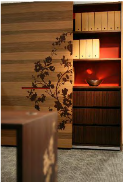
Wall panel with inlaid walnut using laser-cutting techniques. Reverse image used on the desk.
